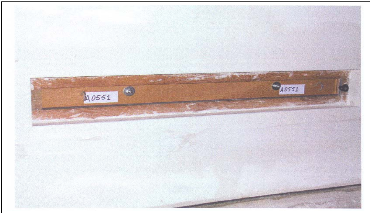
Fig. 10 - Specimen with sealing gasket driven down in closed position (observe on the right the wedge-shaped drive device plugged in ) . Picture taken from the receiving side
